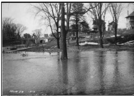
Flooding, North Toronto, 29 March, 1916. CTA
